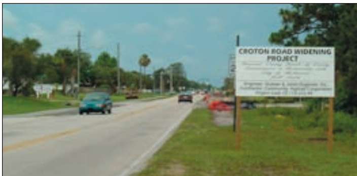
Looking south on Croton Road just north of Lake Washington Road in Melbourne.
